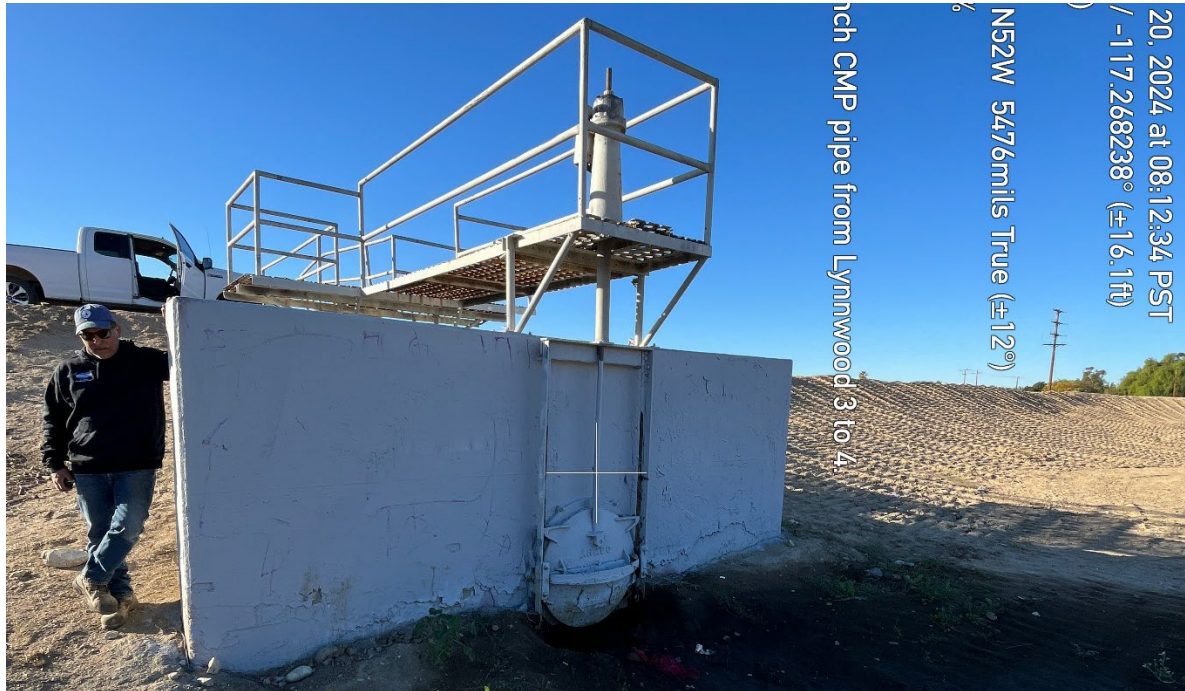
Figure U- Slidegate over outflow in forefront of drop-inlet structure typical for Lynwood Basin Nos. 2 and 3
