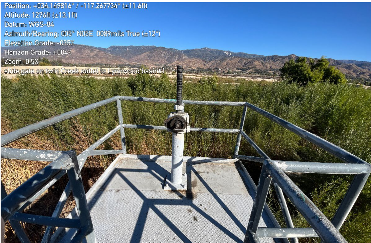
Figure S - Twin Creek Recharge Basins Drain-Gate Mechanism
