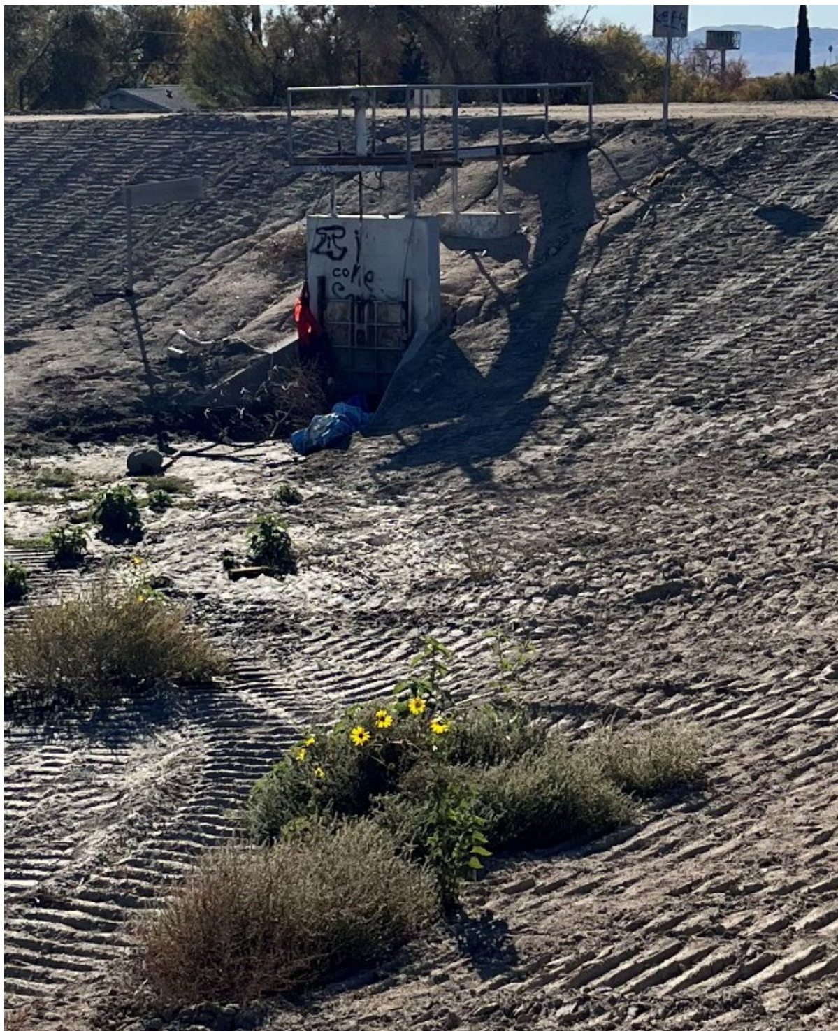
Figure T- Lynwood Basin No. 1: 48-inch diameter slidegate over outlet – observed in full open position Nov. 20, 2024
