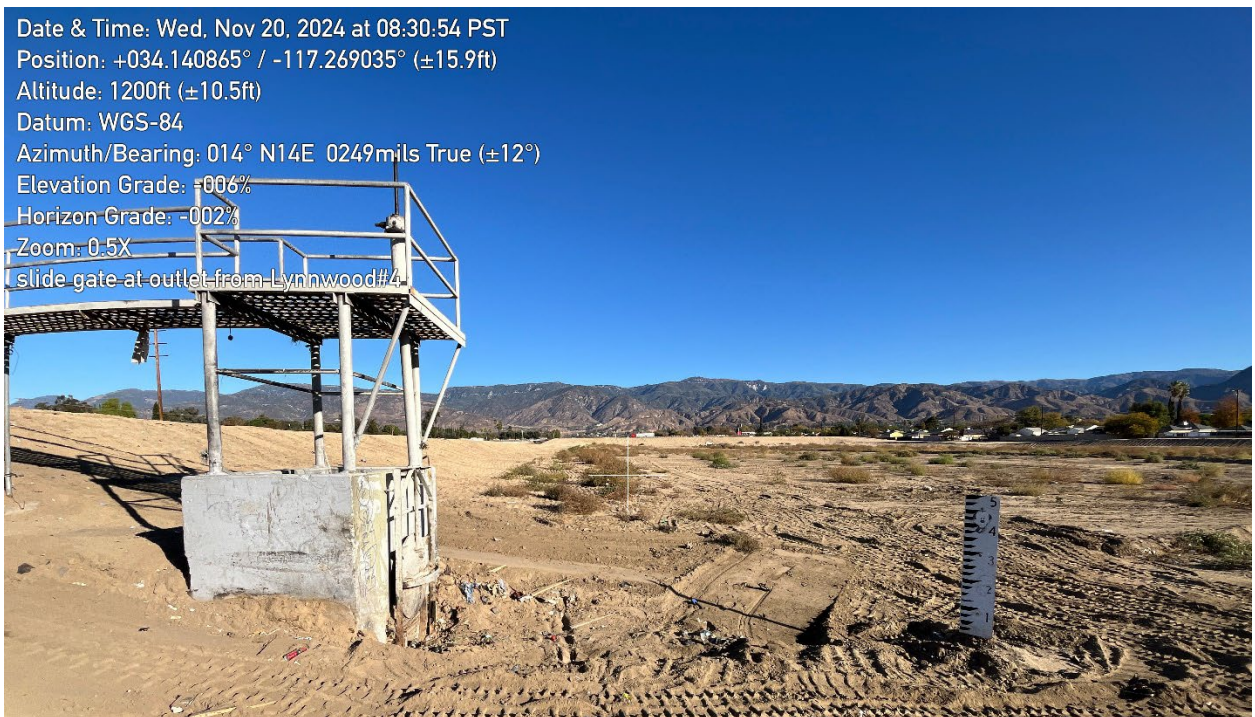
Figure X - Lynwood Basin No. 4 36-inch diameter Slidegate over outlet pipe - Observed open on Nov. 20, 2024
