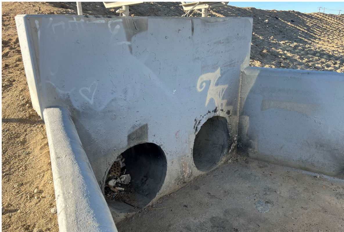
Figure V - Sidewall of drop inlet to dual-pipe outflow culvert at Basin Nos. 2 & 3 (picture where man was standing)
