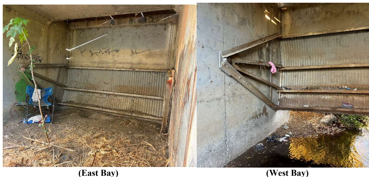
Figure 2.1 – Existing Conditions of Radial Gates at WCDC Diversion Structure No.1C
