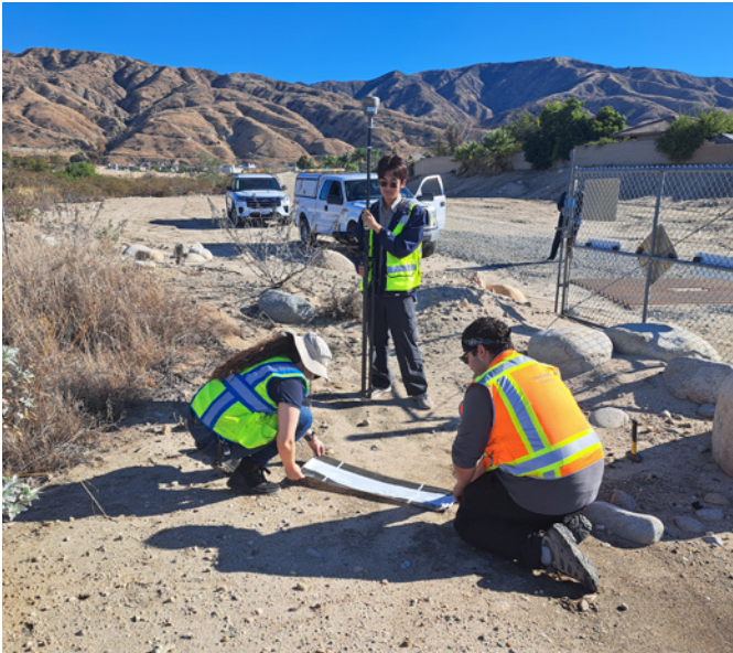
Students from Cal Poly Pomona conduct a survey at the proposed Oak Creek recharge site assisted by the Westland Group engineering firm. Photo Credit: Oak Creek Water Conservation Group
